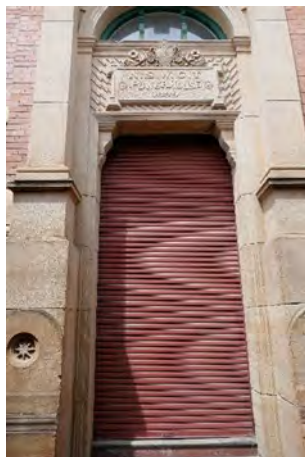
Figure 9 The original entry has been infilled with a roller door: note decorative spandrel panel
