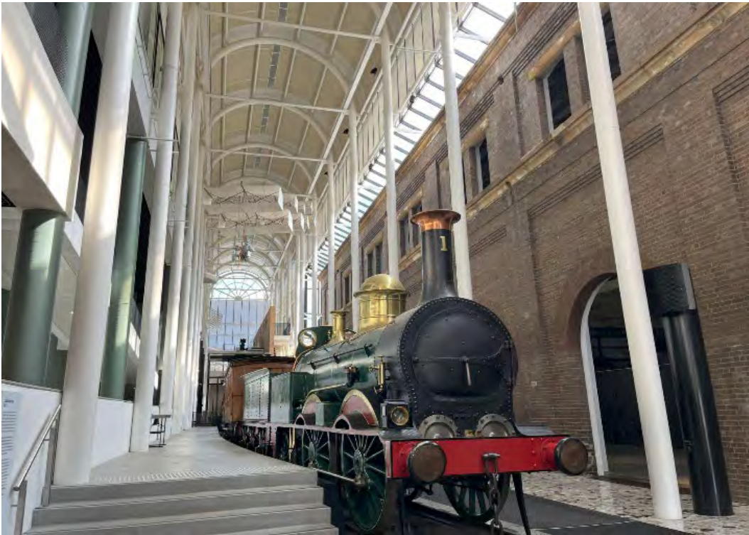
Figure 32 View looking north through Vault 1: Locomotive No 1 is in the foreground and the west elevation of the Turbine Hall is at right
