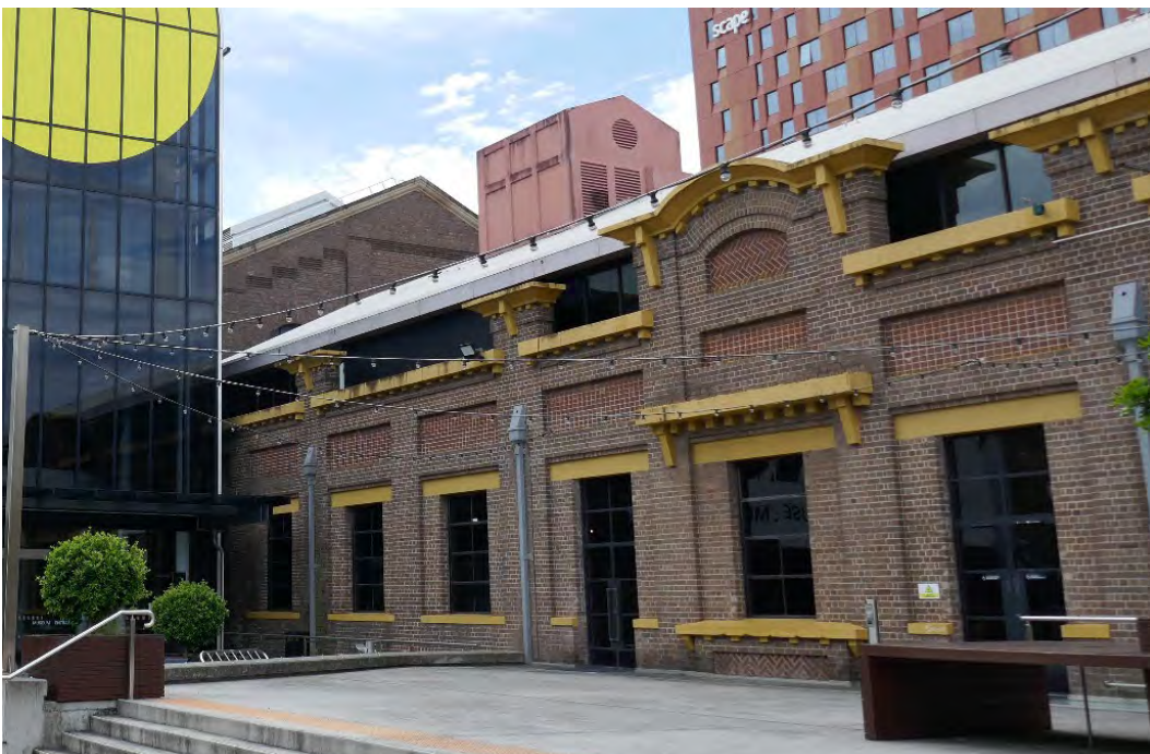
Figure 21 View of the Switch House (right) from the Harris Street Forecourt
