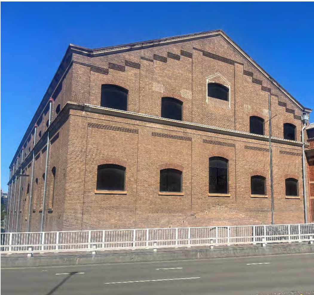
Figure 3 North and east (part) elevations of the Boiler House as seen from William Henry Street
