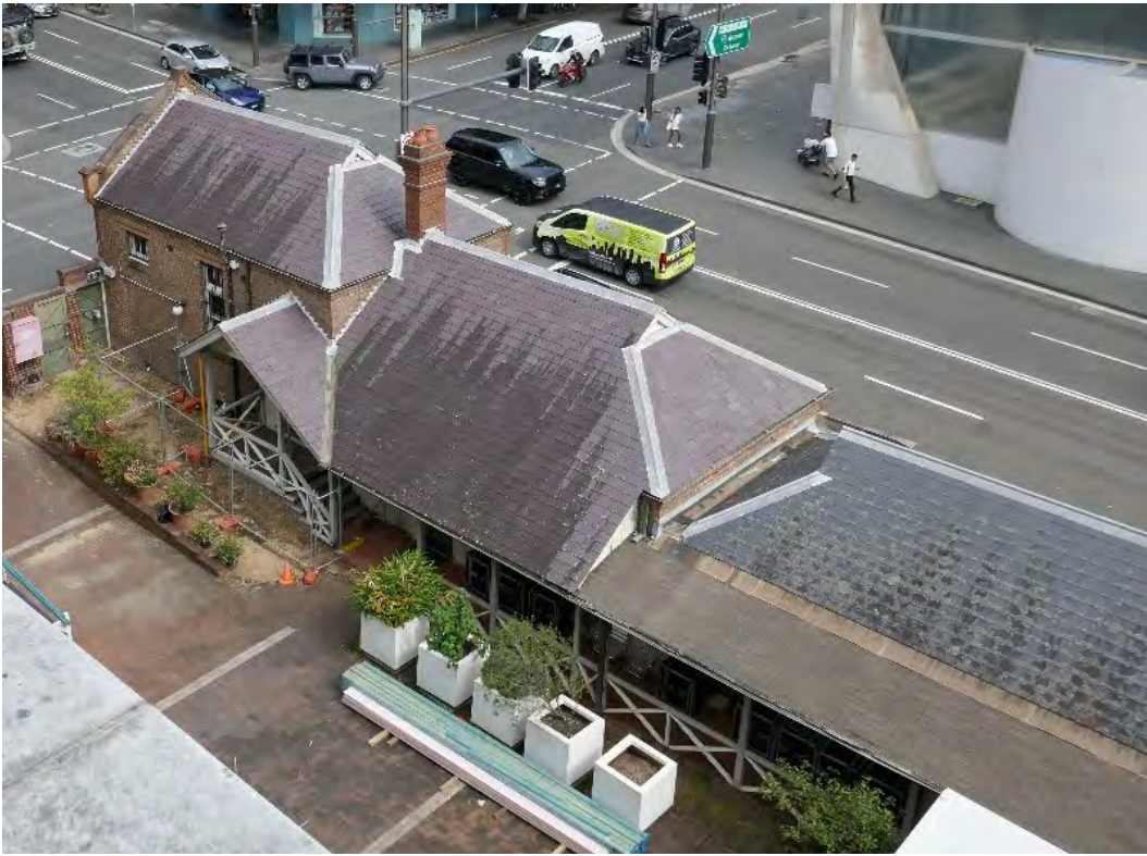
Figure 15 Elevated view of the rear (south) elevation of the Post Office
