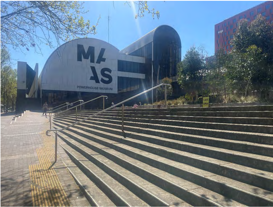
Figure 42 Steps leading from Harris Street up to the forecourt (September 2023)
