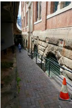
Figure 8 Paved laneway to the north
