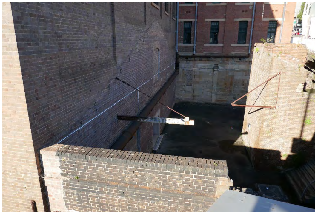
Figure 11 View looking west into the Pump house remnants from William Henry Street: note the chimney base at right
