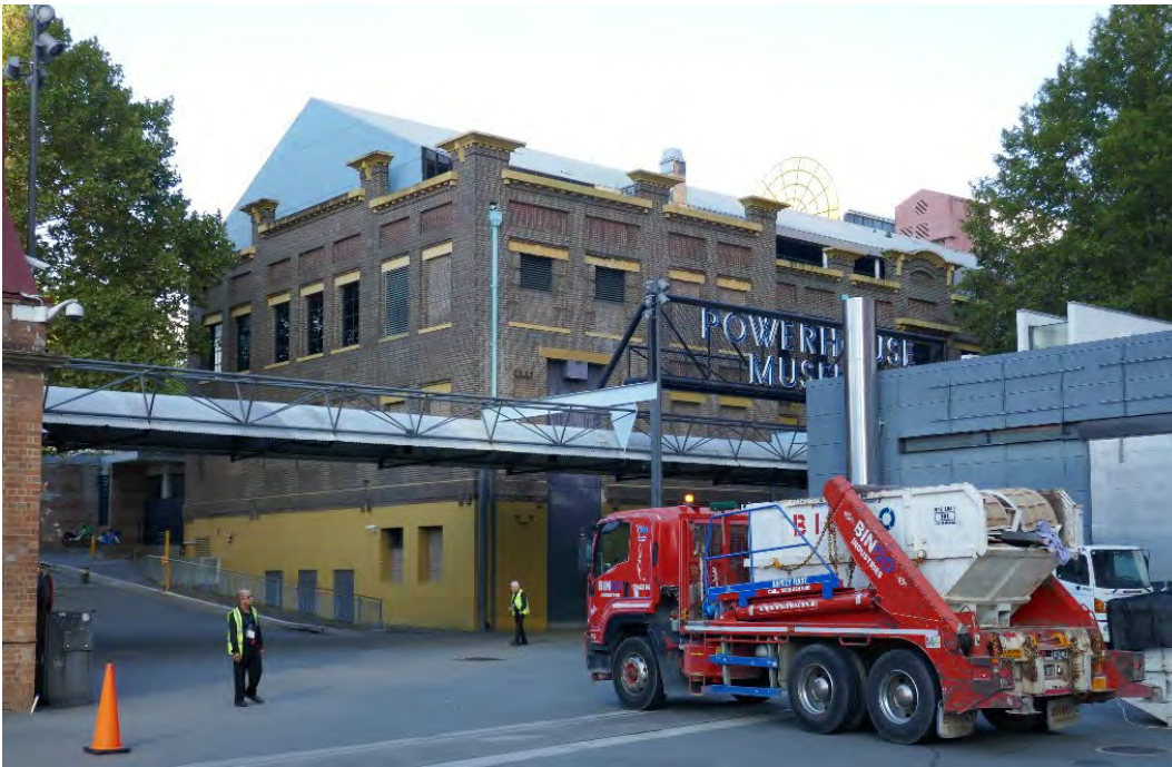
Figure 20 South and east (part) elevations of the Switch House
