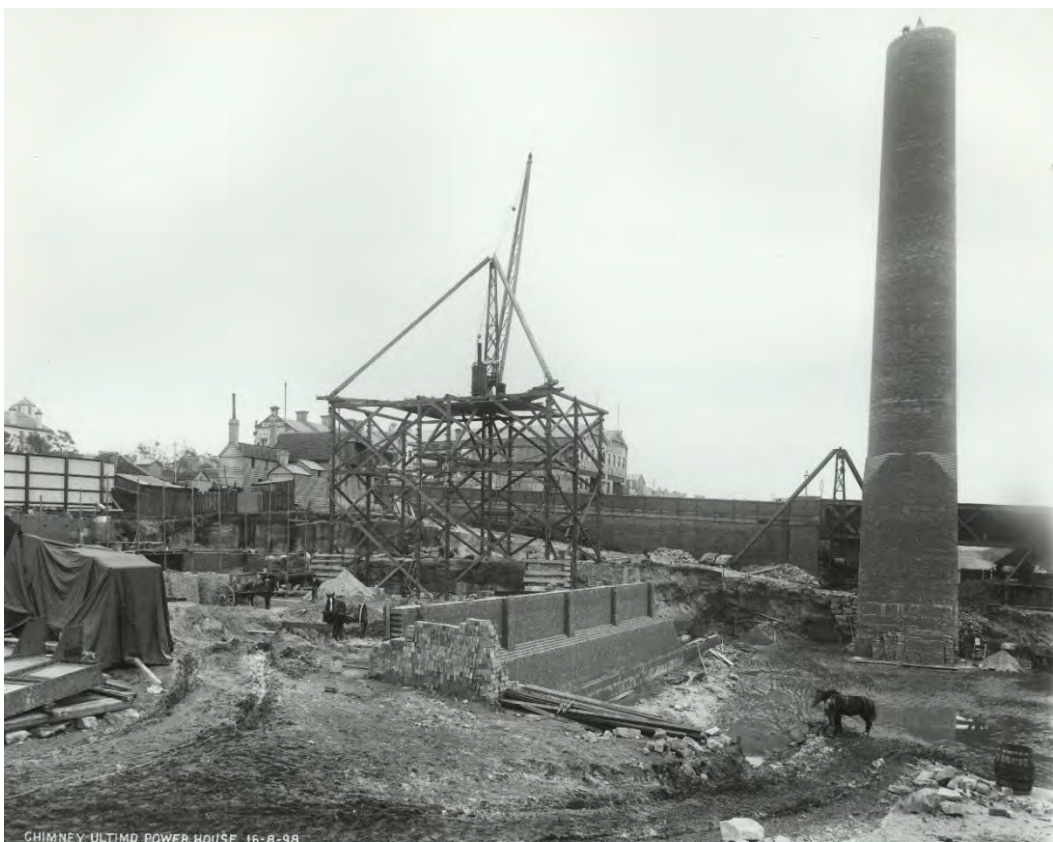
Figure 5 Power House under construction, c. 1898: view looking north to the pump room and stack
