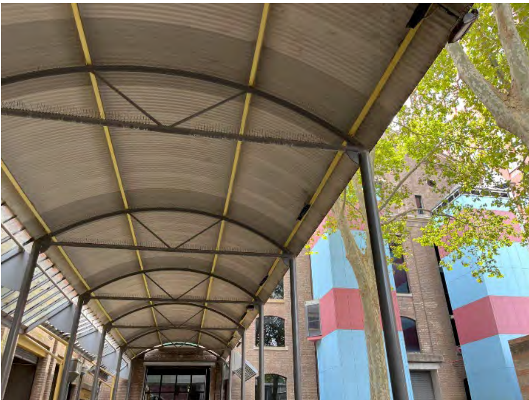
Figure 44 View from the covered walkway looking north towards the Boiler House
